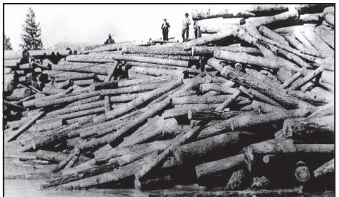
Decked logs waiting for spring run off
