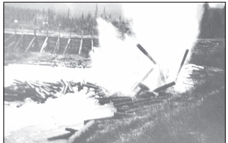
Using dynamite to break log jam
