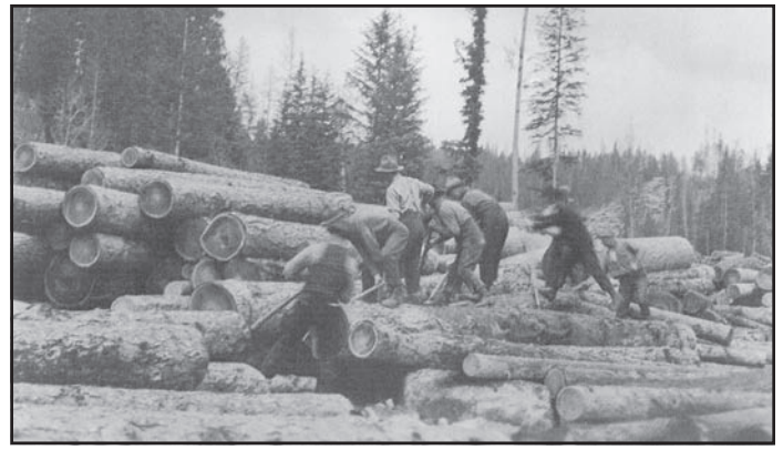
Breaking the decks
